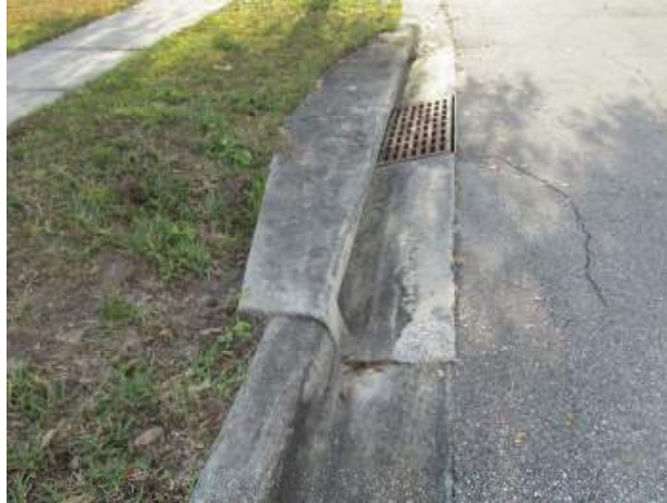
Severe settlement behind catch basin
