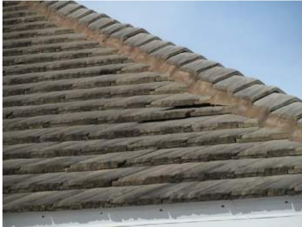
Concrete tile roof with loose tiles
