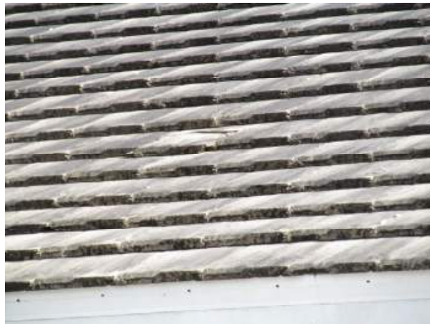
Concrete tile roof with broken tile
