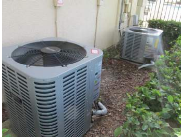
Condensing units for split systems
