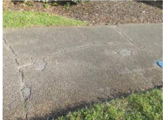
Asphalt pavement walkway with block cracks
