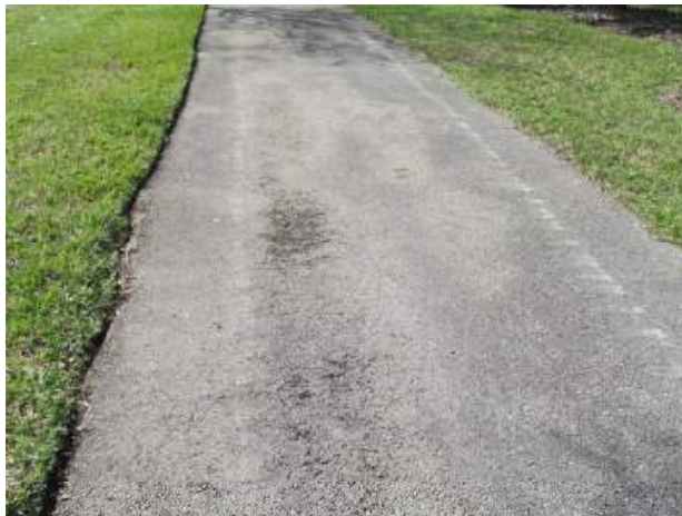
Asphalt walking path with surface deterioration
