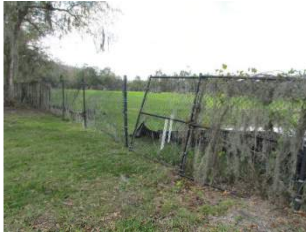
Chain link fence with lean evident
