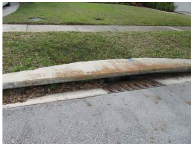
Severe settlement behind catch basin
