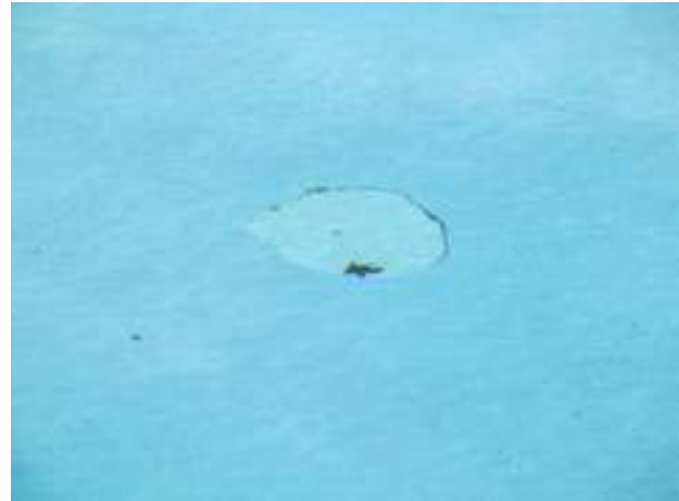
Missing plaster evident
