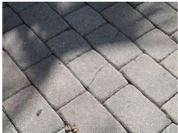
Masonry pavers with isolated cracks evident
