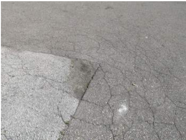
Asphalt pavement with alligator cracks
