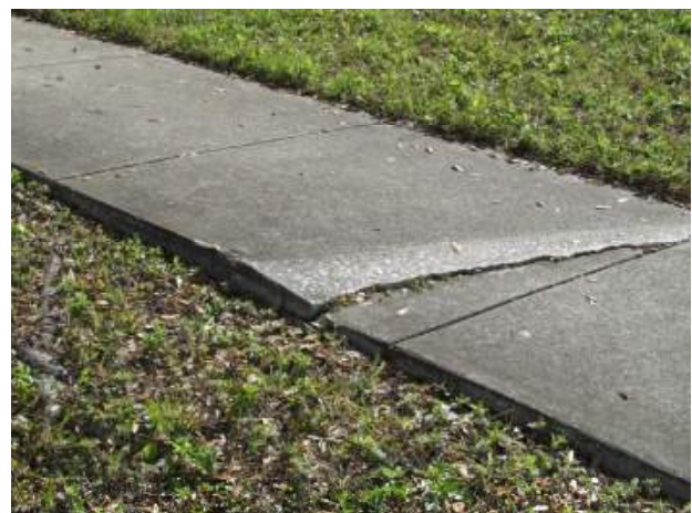
Concrete sidewalk with cracks and trip hazard
