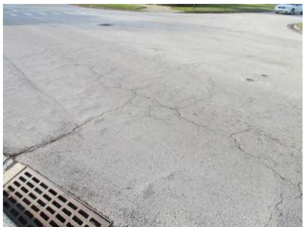
Asphalt pavement with alligator cracks and shoving
