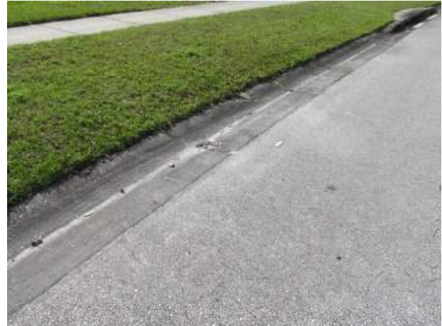
Concrete gutter with cracks
