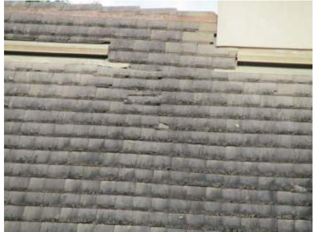
Concrete tile roof with broken tiles
