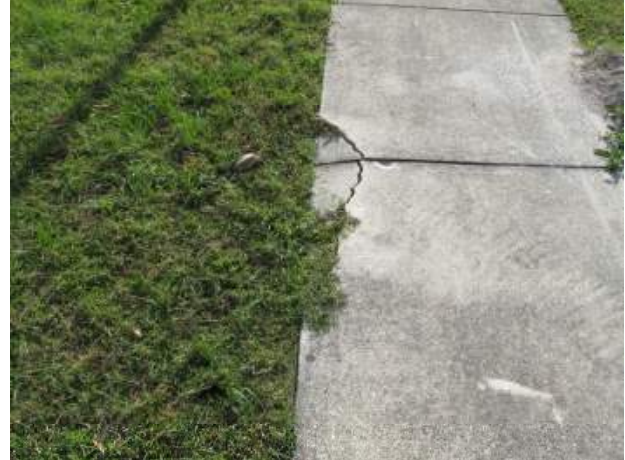
Concrete sidewalk with cracks
