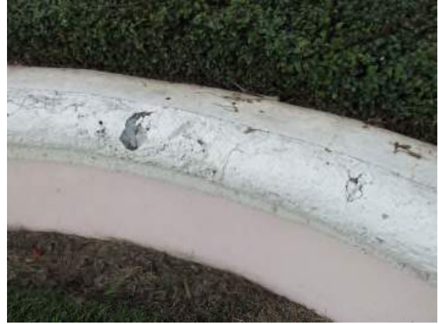
Coping damage at entrance signage
