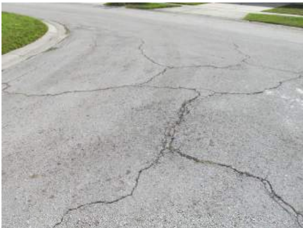
Asphalt pavement with block cracks
