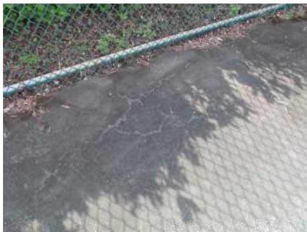
Hairline cracks evident
