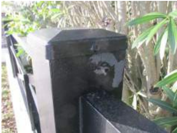
Finish deterioration at bridge railing
