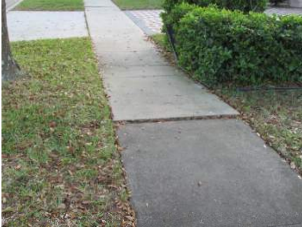
Concrete sidewalk with trip hazard
