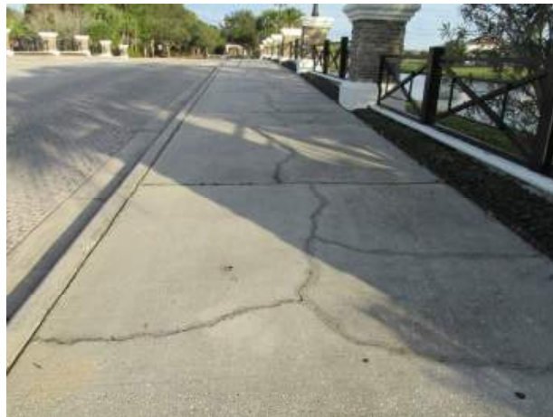
Concrete sidewalk with cracks
