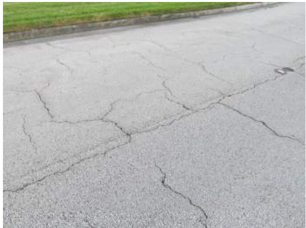
Asphalt pavement with severe block cracks
