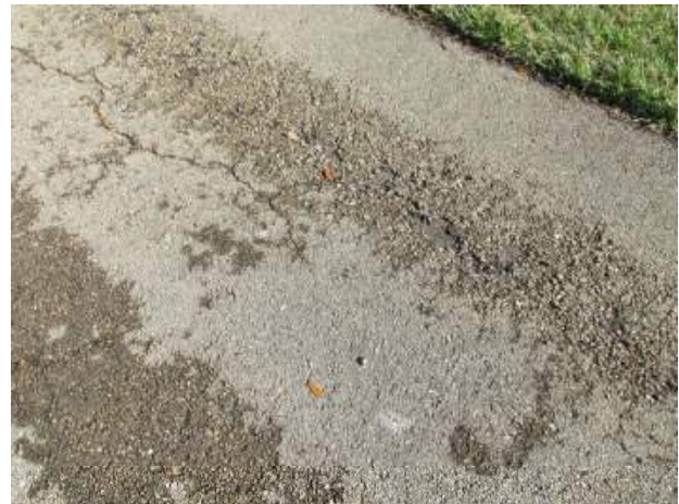
Asphalt walking path with surface deterioration
