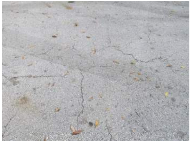
Asphalt pavement with alligator cracks
