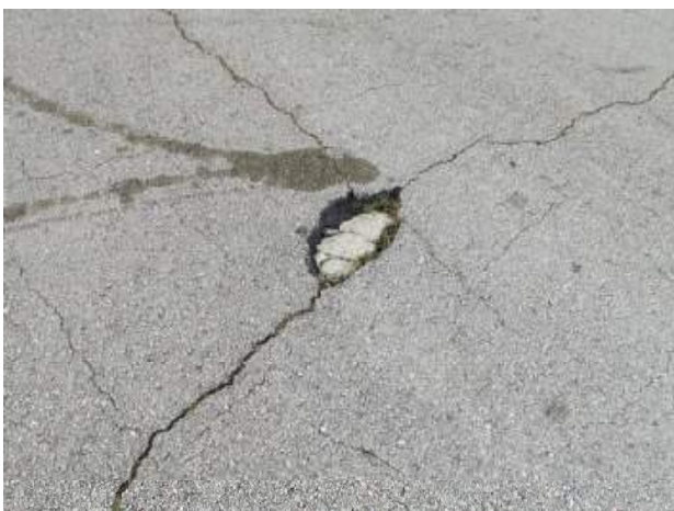
Asphalt pavement with pot hole
