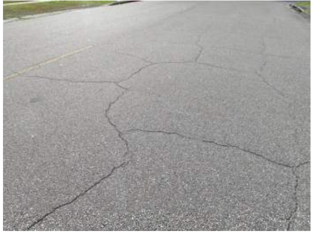
Asphalt pavement with block cracks
