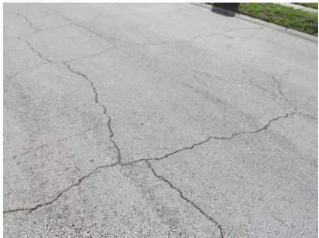
Asphalt pavement with block cracks
