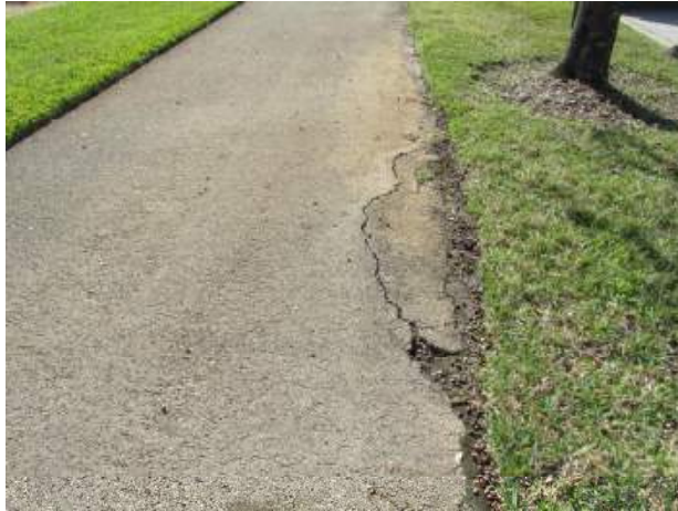
Asphalt pavement walkway with edge cracks
