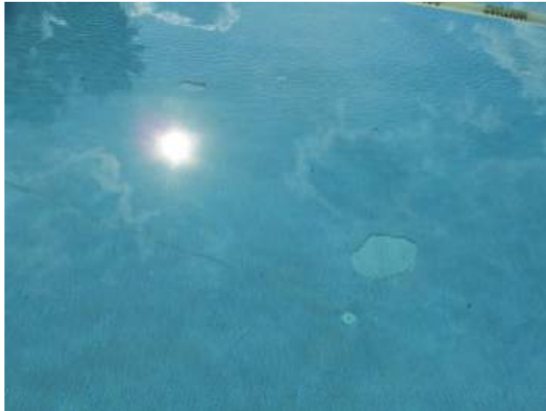
Missing plaster evident
