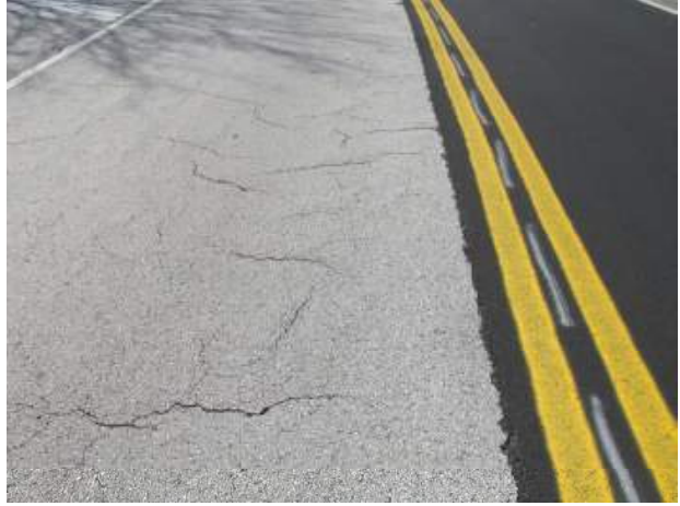
Asphalt pavement with slippage cracks
