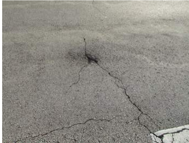
Asphalt pavement with pot hole
