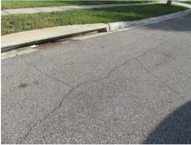
Asphalt pavement with block cracks
