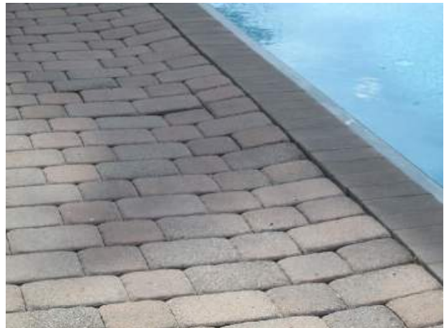
Deck pavers with isolated settlement evident
